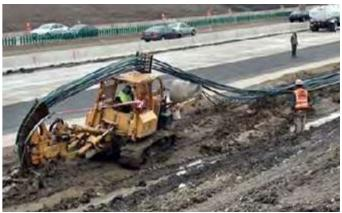
• When new roads are constructed or rebuilt, HDPE conduit is one of the first utilities to be installed, often for future fiber optic cable ("Dig once")
