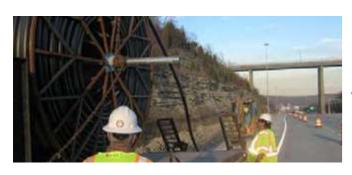
HDPE conduit protects fiber optic & copper communication cables and power cables
